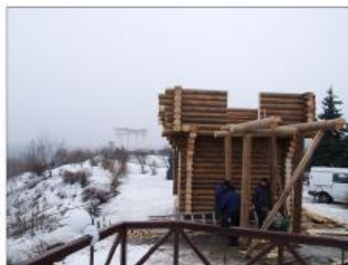
Fig. 7. Construction of the Podilska tower, February 05, 2009; photo by K.Y. Trehubov.
