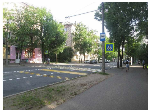
Fig. 1. The typical example of the hump's installation in Minsk, Belarus
